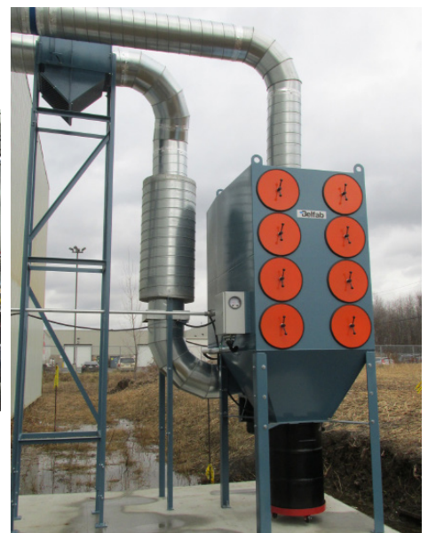
INDOOR PLASMA MANUFACTURING AREA CONNECTED TO AN OUTDOOR H8 CARTRIDGE DUST COLLECTOR
