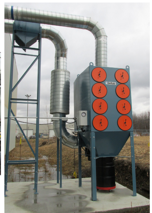
INDOOR PLASMA MANUFACTURING AREA CONNECTED TO AN OUTDOOR H8 CARTRIDGE DUST COLLECTOR
